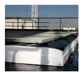
The insulation boards are loose laid over the weatherproofing, there is no requirement to adhere or mechanically fix the boards. Jablite Filter Membrane and gravel ballast and/or paving slabs are used to secure the insulation to the deck.
